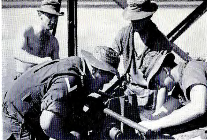
New Zealand army engineers work with Vietnamese to repair a bridge north of Saigon.
